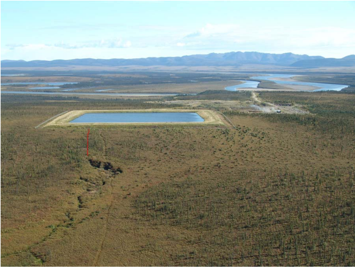
Photo 1: Kiana has had problems with a breaching of the sewage lagoon, August 29, 2007.
